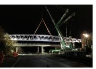
Warren truss bridge at Tithebarn, Exeter being craned into place over the M5
